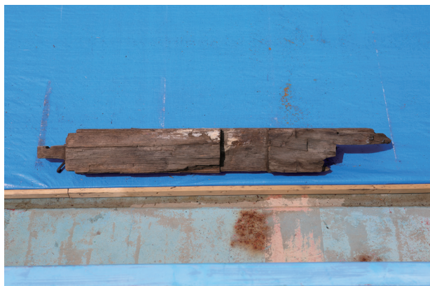
図3a 保悪部材 Fig. 3a Building material in poor condition
