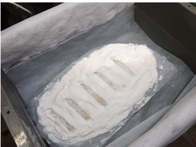
図5 表面を石膏で保護して行う脱塩処理例 Fig. 5 Example of desalination treatment employing surface protection by applying plaster
