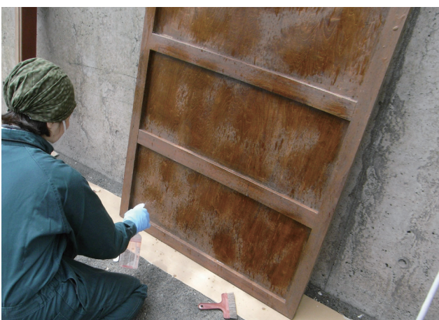
図9 洗浄後、裏面に防カビ剤TBZを塗布 Fig. 9 Post-washing application of anti-mold agent TBZ to the back side
