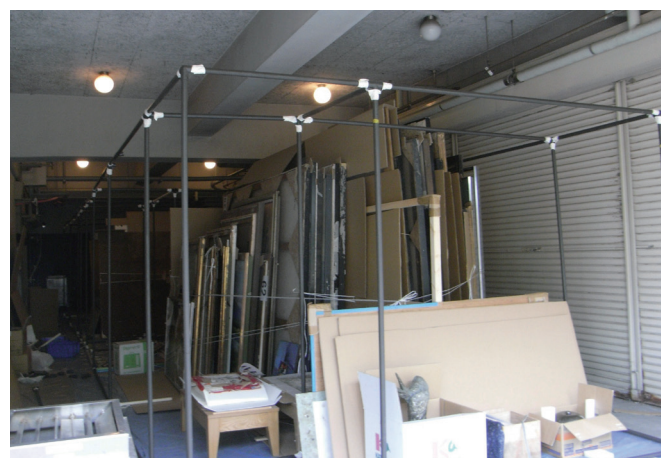
図10 ビニルシートで覆う被覆燻蒸のための鉄骨。カビの繁殖がひどいため処置作業前に燻蒸を行った。 Fig. 10 Steel frame to hold up the vinyl sheet for fumigation using a vinyl sheet. Pre-treatment fumigation was necessary because of extensive mold growth.
